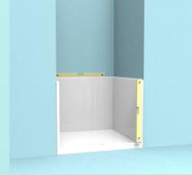
Place the tray section of the Neptune Bathing shower in position and check for Level horizontally from left to right and check for Plumb vertically.
